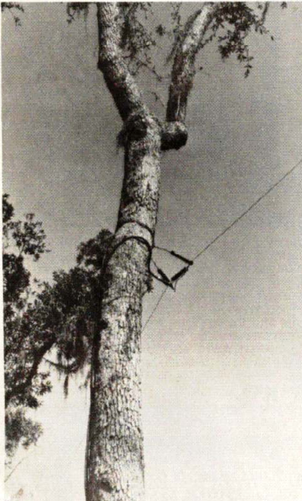
Completed antenna mounted in tree.
